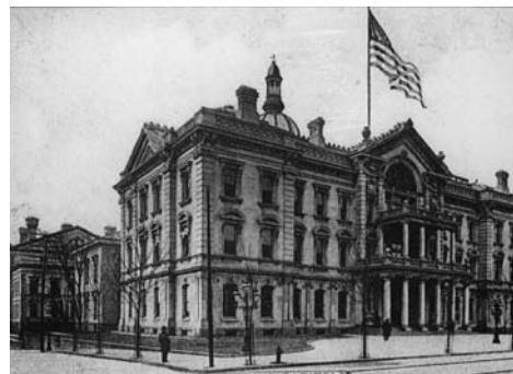
North and Northeast Facades, c.1905 Major reconstruction took place after a devastating fire in 1885.
