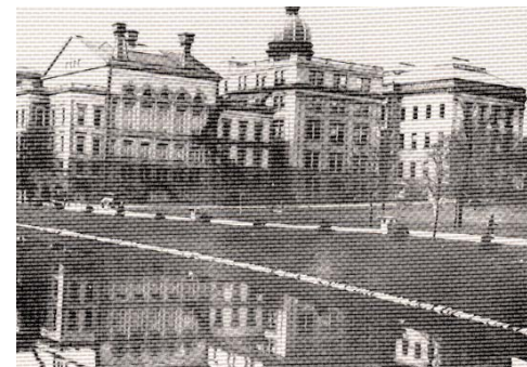
South and East Facades, c.1912-17 The building remained nearly unchanged until current renovations began in 1986.
